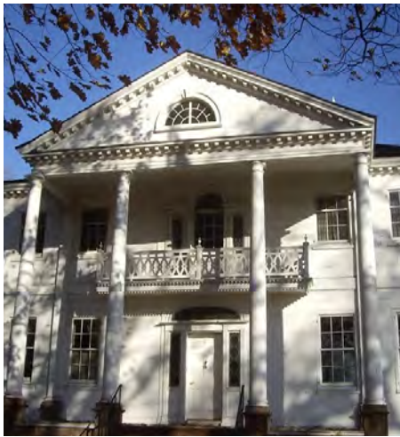
Restored portico and pediment, supported by grand Tuscan columns
