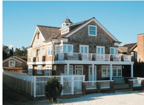
Exterior View Front
